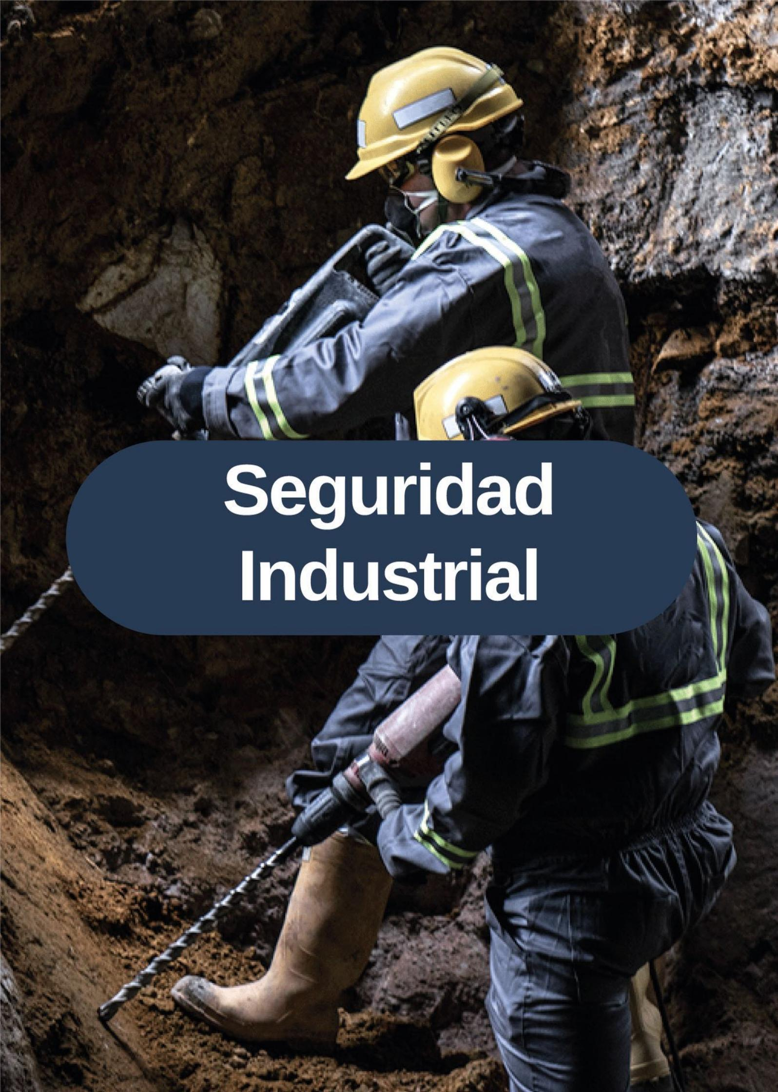
The image shows two workers in a dark, rocky tunnel. They are wearing dark grey protective suits with reflective yellow-green stripes, yellow hard hats, and safety glasses. One worker in the foreground is using a pneumatic drill with a long, twisted drill bit. The background shows the rough, uneven walls of the tunnel.
